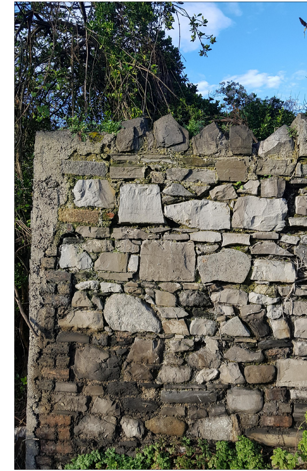
TYPICAL IMAGE EXISTING STONE WALL TO BE RETAINED
