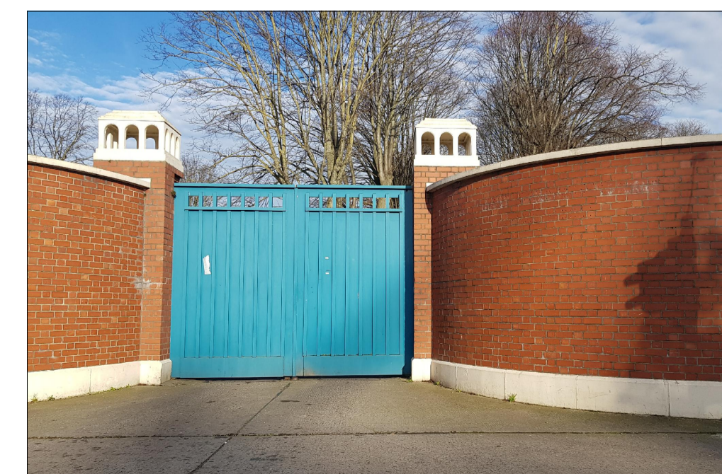
TYPICAL IMAGE EXISTING BRICK WALL TO BE PARTLY REMOVED
