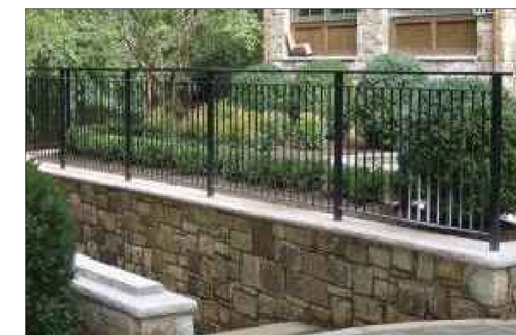
TYPICAL IMAGE RETAINING WALL + RAILING
