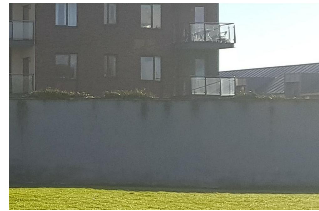
TYPICAL IMAGE EXISTING BLOCK WALL TO BE RETAINED
